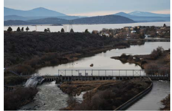
Link River Dam
